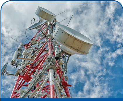
Telecom -Data Infrastructure
